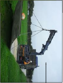
track-way system being laid
